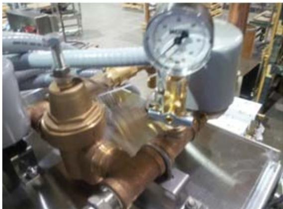
Showing pressure reducing valve for final rinse & gauge\*
